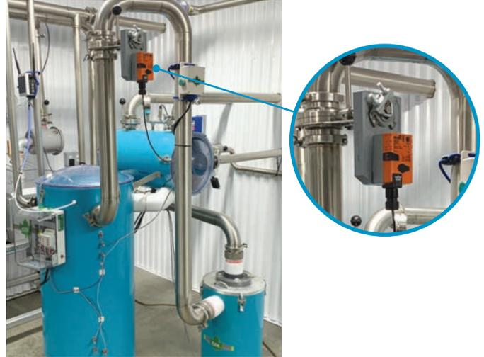
The vacuum protection valve safely prevents sap overflow in your moisture trap or your vacuum pump without shutting vacuum down.
